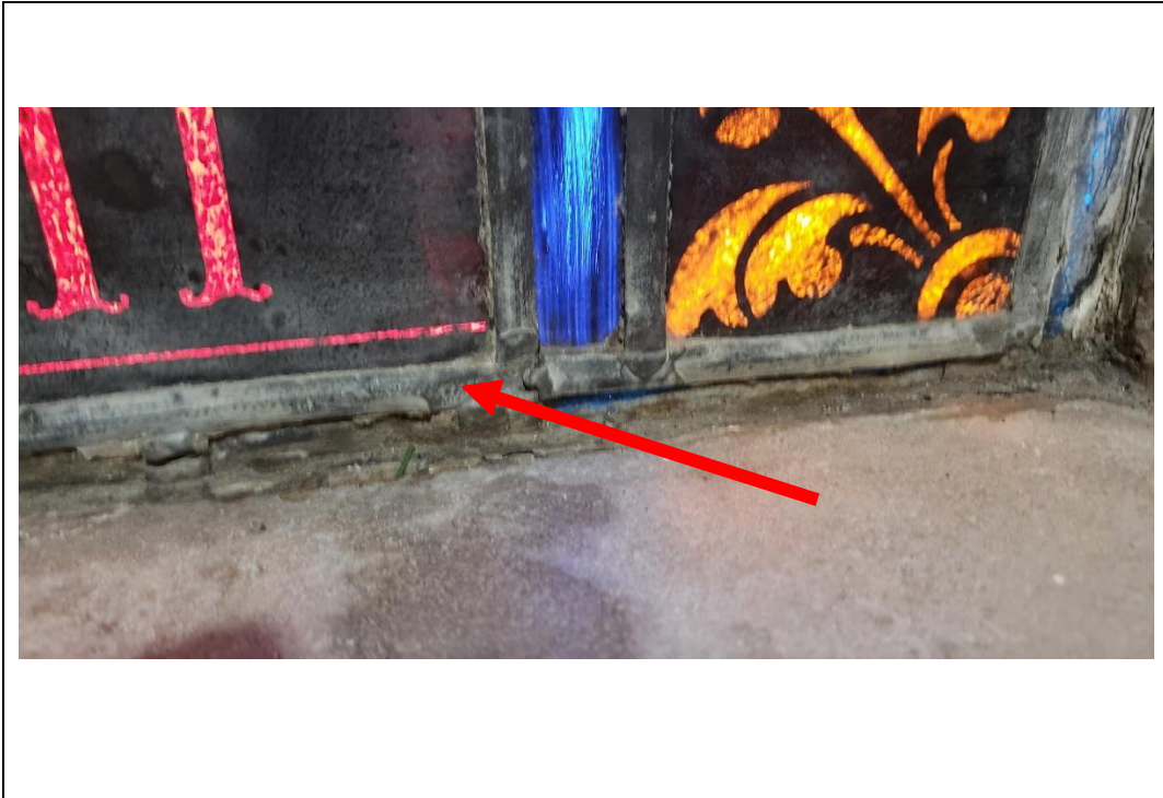
Typical ACM Window Caulk Location (Interior)
