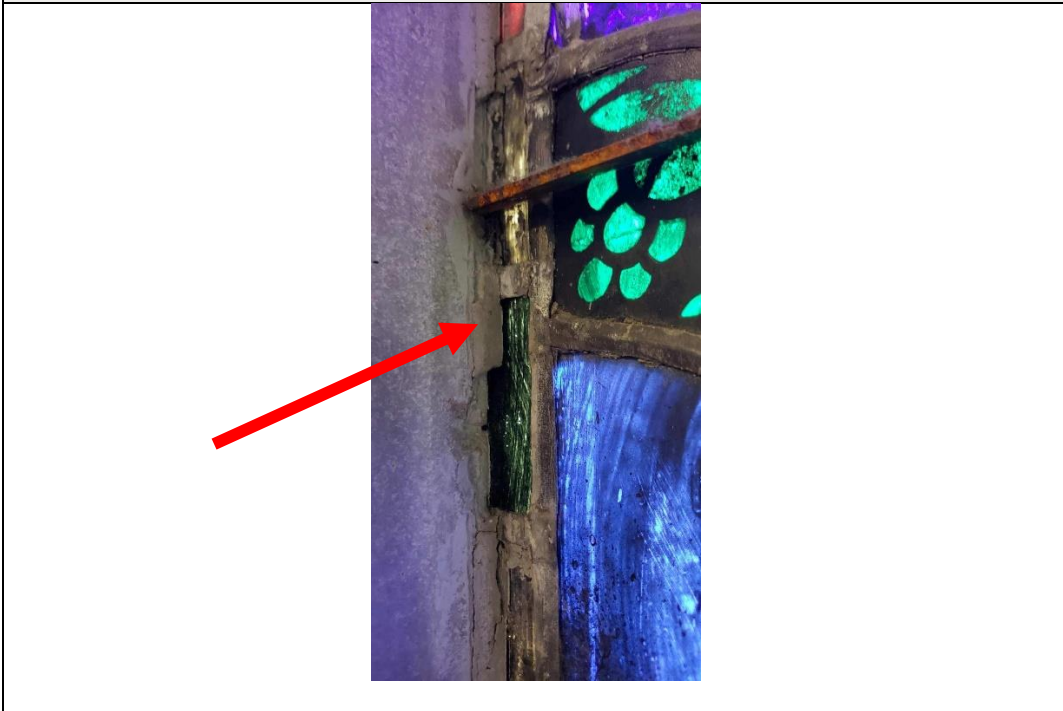
Typical ACM Window Caulk – Sample Location (Interior)
